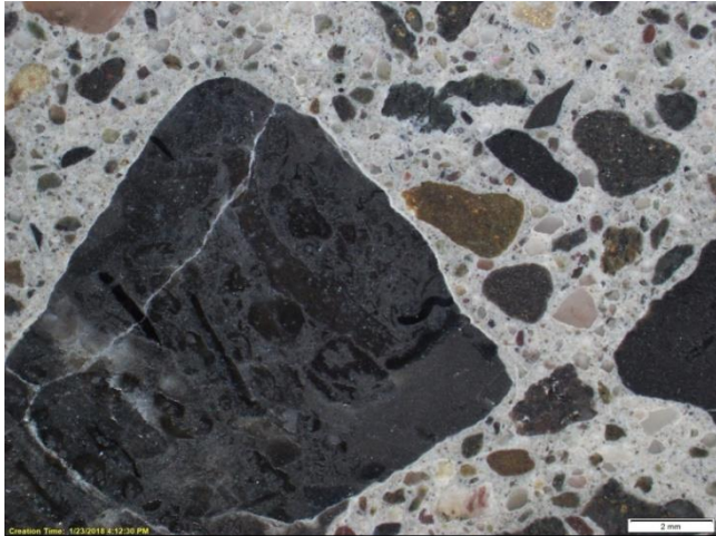
Cut and polished concrete showing white ASR gel filling a crack in a coarse aggregate particle; magnification x8.
