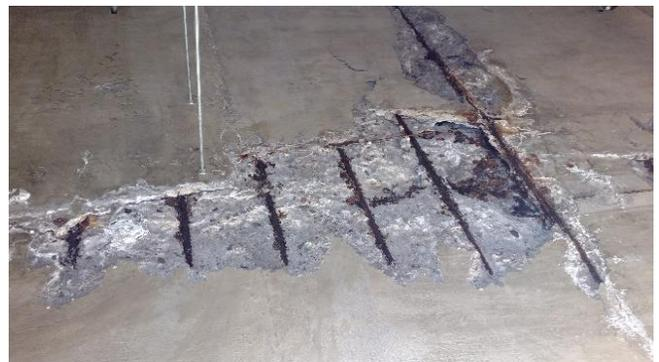
*Slab delamination due to reinforcement corrosion*
