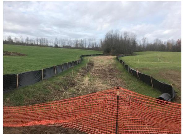
*Proper Construction Sequence: Silt fence installation adjacent to wetland prior to soil disturbance activities*
