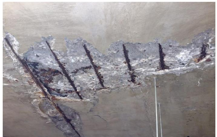
oxidation and corrosion due to the formation of secondary products such as iron oxide (rust) which causes the surrounding concrete to expand, crack, and ultimately fail.
