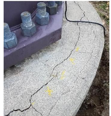
Failing concrete in a caisson foundation
