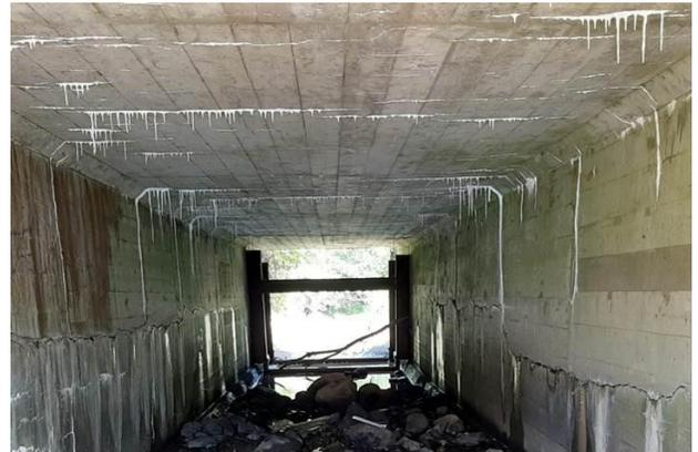
Box culvert with cracking and efflorescence caused by ASR
