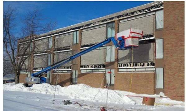
Use of aerial lift for elevated gridding operations of exterior wall tar.
