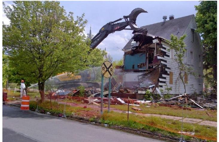
Example of a demolition with asbestos in-place for a vacant residential building.
