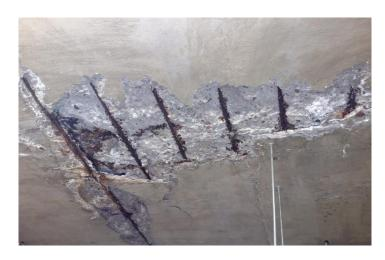
oxidation and corrosion due to the formation of secondary products such as iron oxide (rust) which causes the surrounding concrete to expand, crack, and ultimately fail.
