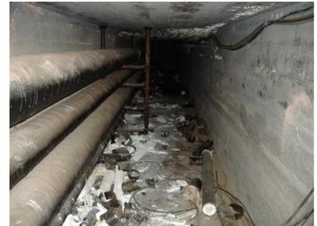
Example of an incidental disturbance of asbestos-containing pipe thermal system insulation (TSI).
