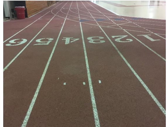
Mercury containing indoor track flooring.
