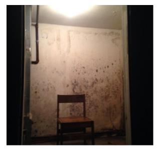
Basements may also be constructed with perimeter drains and/or sump pits that are not fully sealed. Furthermore, as the lowest section of a building, any leaks or flooding from floors above may find a pathway to the basement area, thereby providing another route for water/moisture and possible mold impacts.
