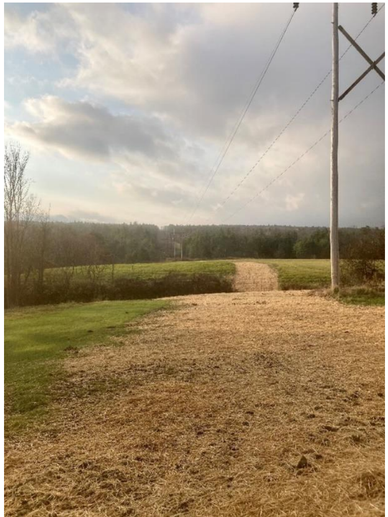
Project access route mulched with straw in preparation for winter conditions.
