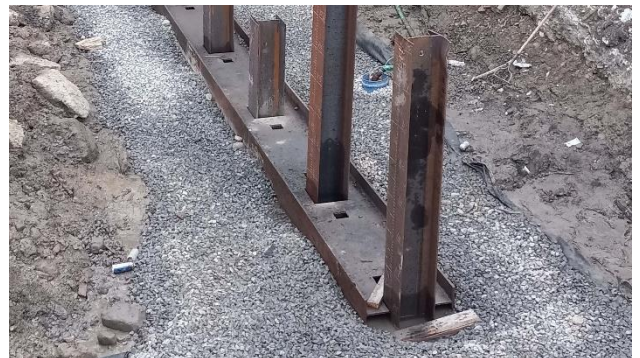
Corrosion of Bridge Abutment Foundation
