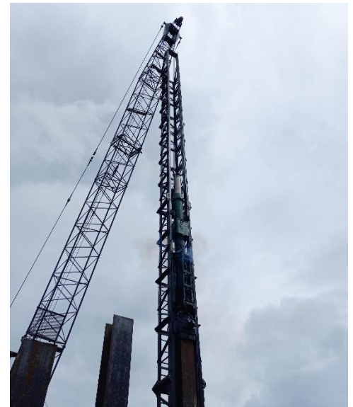
Diesel Impact Hammer
