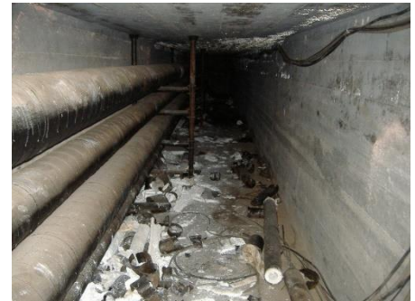
Example of an incidental disturbance of asbestos-containing pipe thermal system insulation (TSI).
