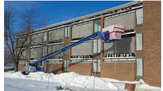
Use of aerial lift for elevated gridding operations of exterior wall tar.
