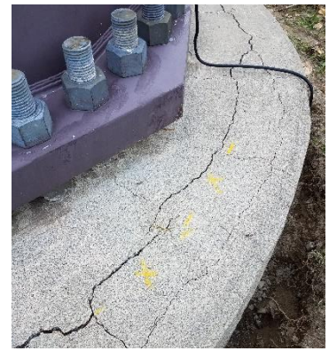
Failing concrete in a caisson foundation.
