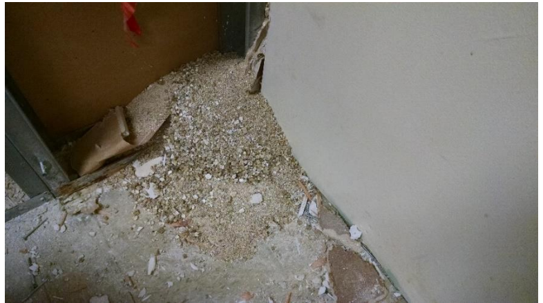
Vermiculite used in wall cavity (above) and floor (below)
