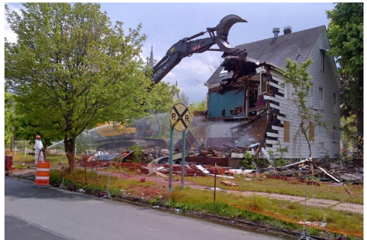
Example of a demolition with asbestos in-place for a vacant residential building.
