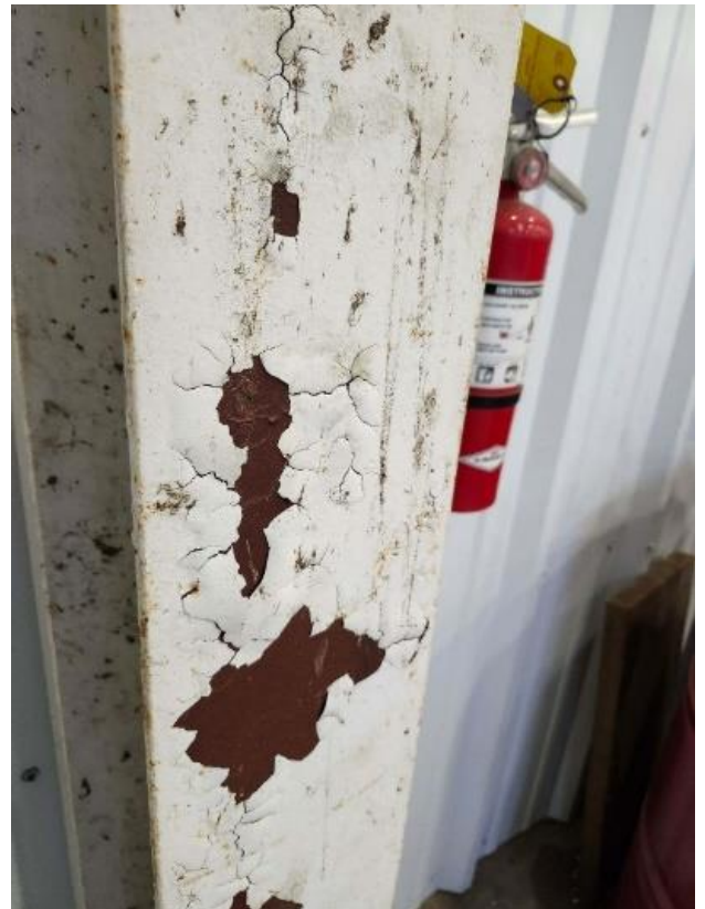
Deteriorating lead-containing paint.
