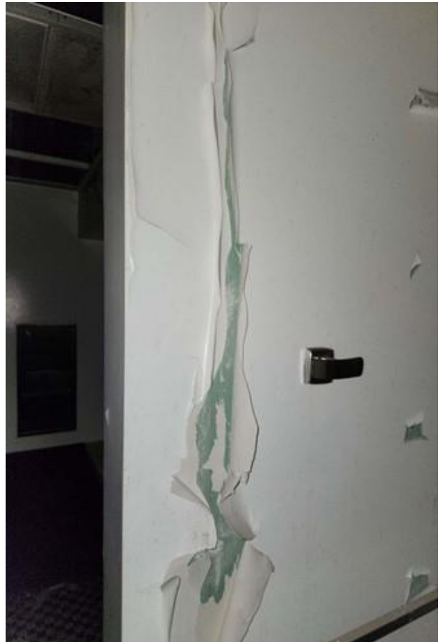
Water-damaged and peeling lead-containing paint.
