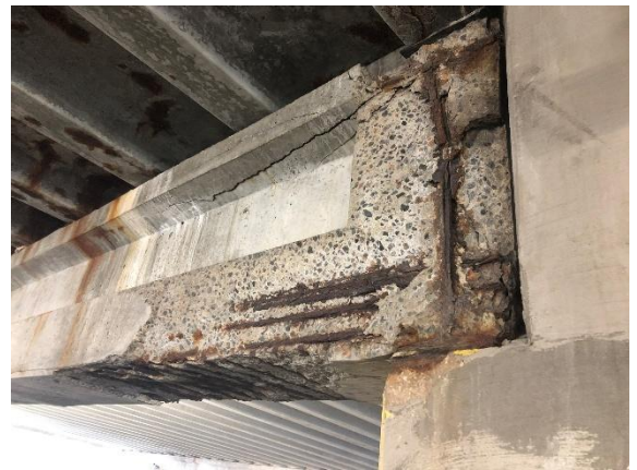
Steel rebar corrosion.
